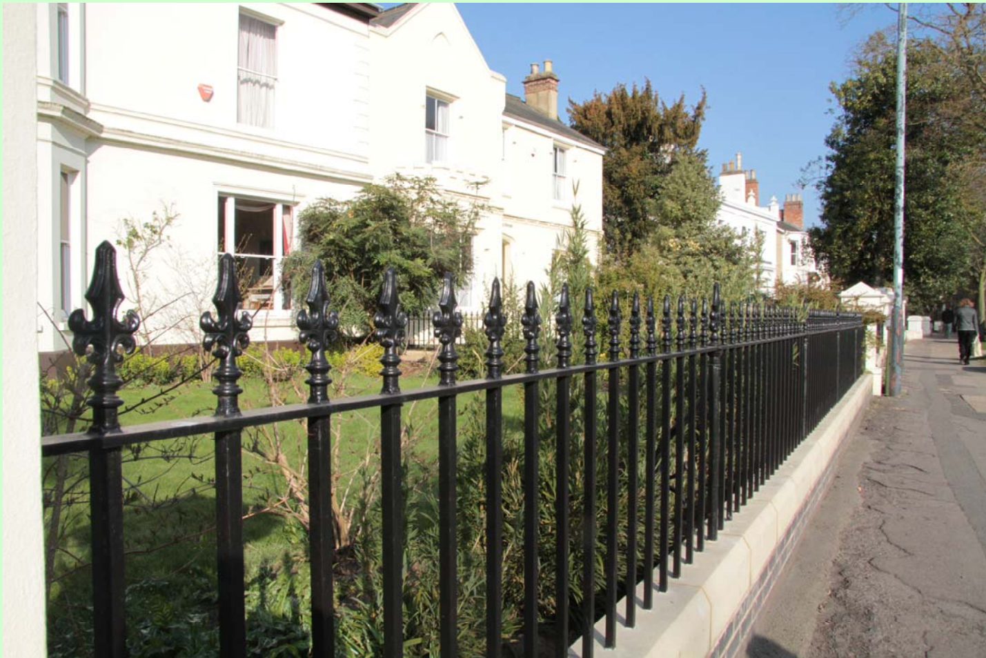
Railings at 30, 32/32a Willes Road
