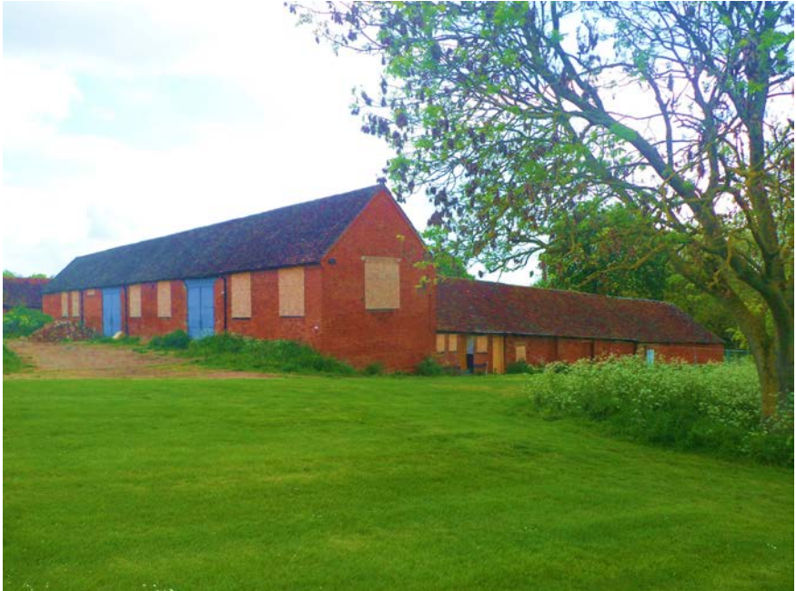
Currently unused buildings
