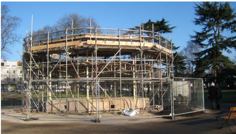
Work in progress on bandstand
