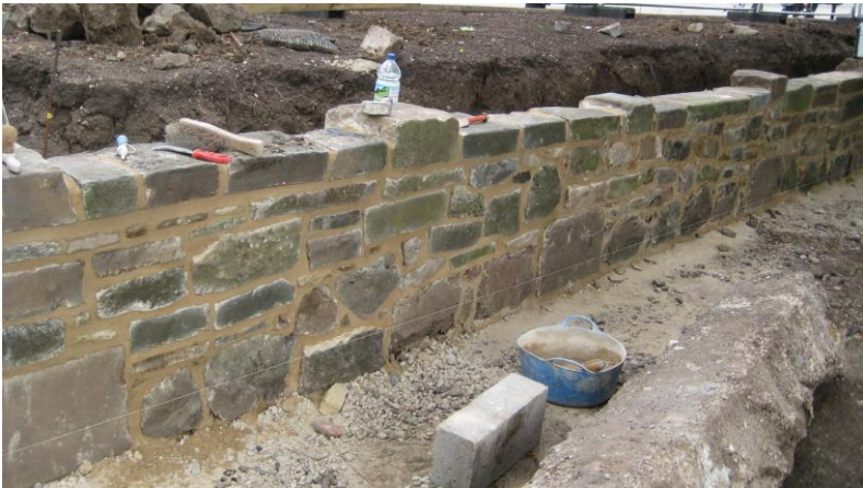
Retaining wall along the Parade being rebuilt
