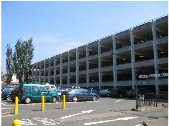
Covent Garden car park
