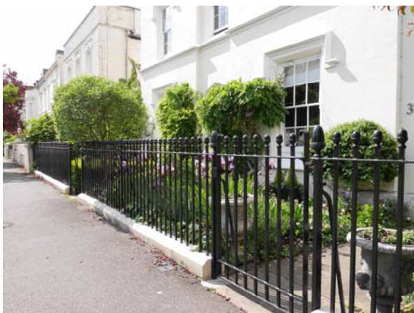
Railings in Russell Terrace
